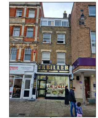
3 FASCIA SIGN PICTURE AFTER WINDOW CANOPIES REMOVED
